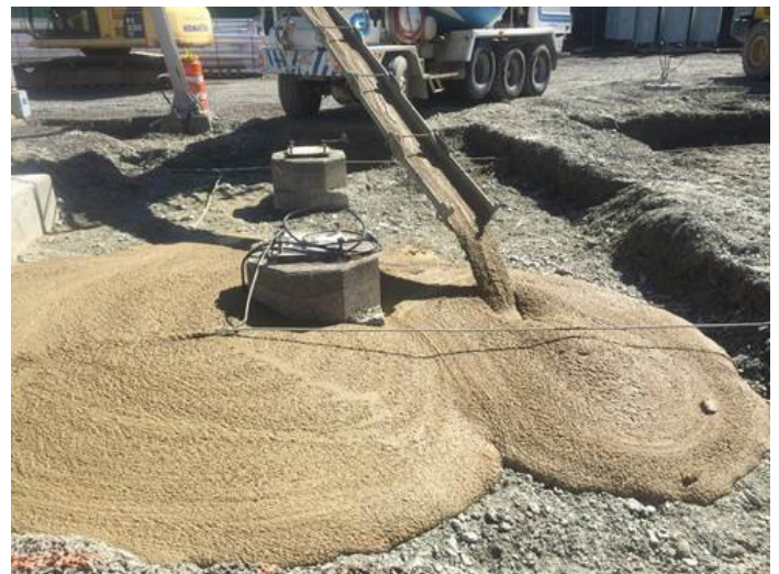
CLSM Placement around Existing Drilled Piers (Structure Upgraded)
